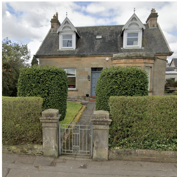
Figure 9.4: Streetview image of 22 Station Road, Broxburn
