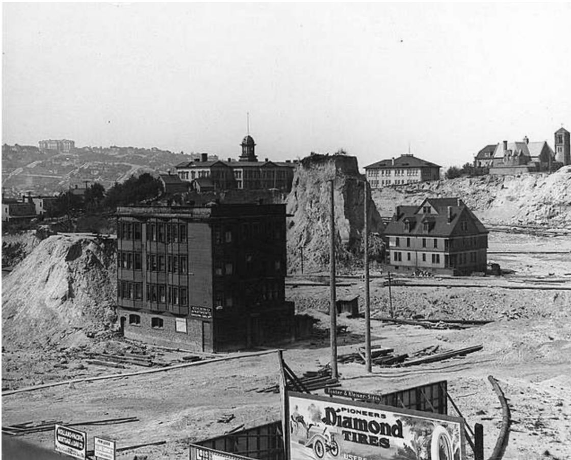
Figure 5.4: Image of the Denny Regrade in Seattle 1910. In the distance on the hill is Queen Anne high school where Wallace would graduate in 1917. Entire hills were washed away into Puget sound between 1908-1911.
